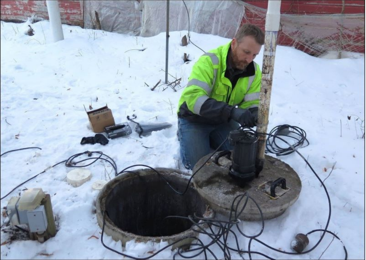
Tim Haeg, a professional septic system designer and installer, works to replace a malfunctioning switch in a septic system in St. Joseph, Minn., on Monday. Kirsti Marohn | MPR News
